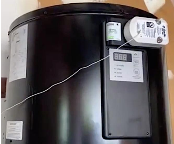
Figure 8. HPWH responsive to KUDL FM in Sacramento, July 7 th 2021
